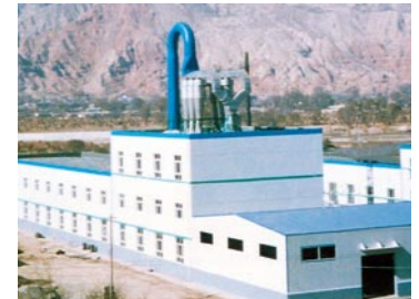
甘肃临洮气流干燥现场 DG Air Stream Dryer in Gansu Lintao
